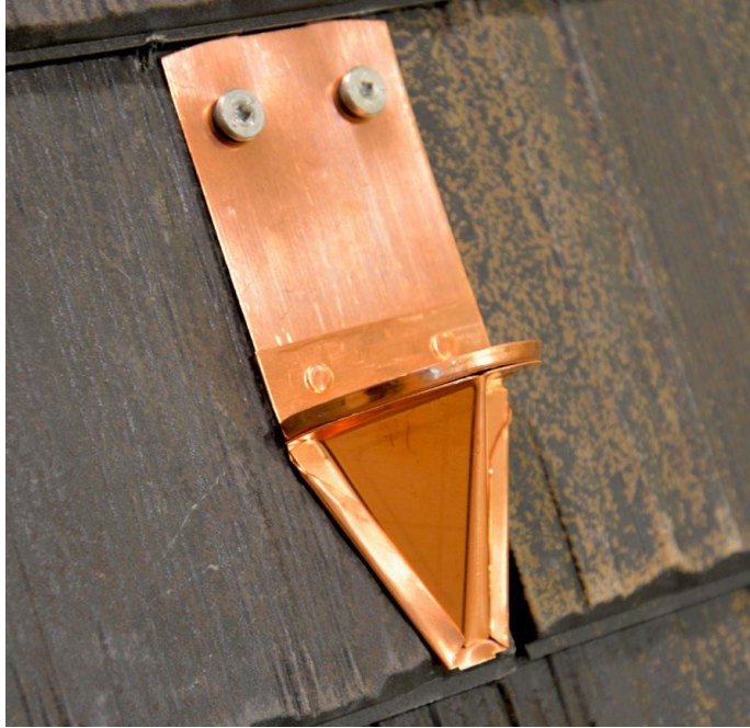
Copper PD30 Snow Guard on F-Wave Hand Split Shake
